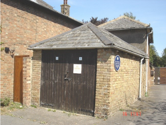
Fire Pump Accommodation
